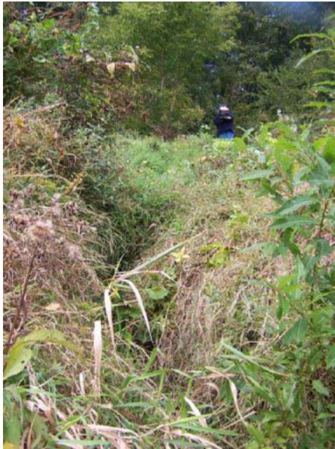
Wickey Site – Gully caused by overland runoff – June 2006
