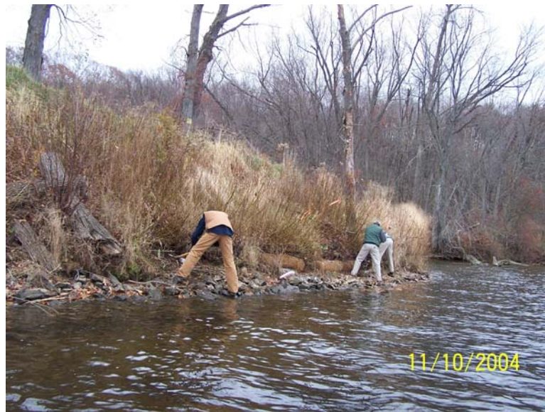
Repair at Shearer Site – November 2004
