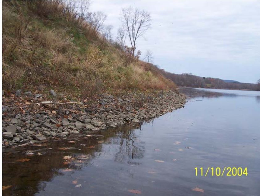
Urgiel Upstream Site Area of Repair - November 2004
