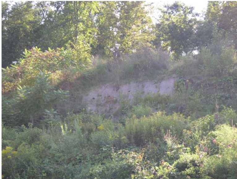
Urgiel Upstream – Eroded/Slumped Bank Face with Bank Swallow Nesting Cavities? – September 2006
