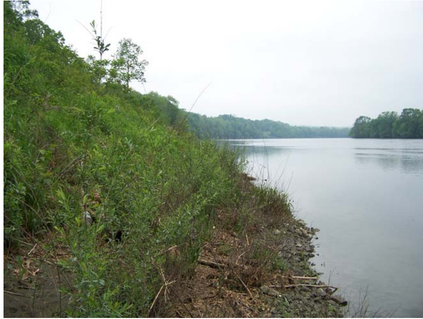
Urgiel Upstream Site Area of Repair – October 2006
