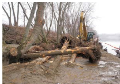
View of the construction of an LWD structure.
