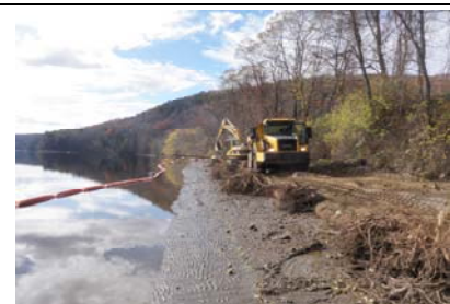
View of the bench and river looking south.
