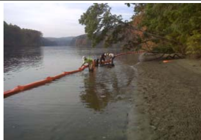
Davenport crews installing the turbidity curtain.
