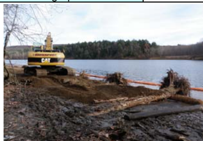
View of the bench construction and large woody debris .
