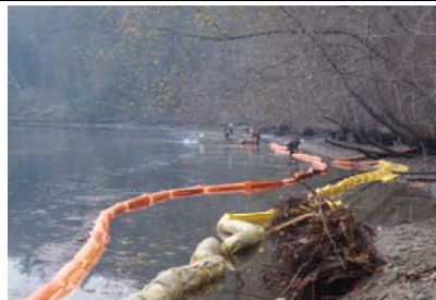
View of the installation of the 8' turbidity curtain.
