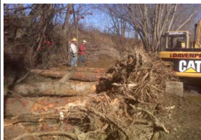
View of the construction of the "scalloped" eroded areas.
