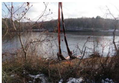
View of the turbidity curtain removal.
