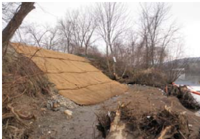
View of the restoration treatment to the access road
