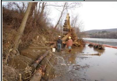
View looking north at the last LWD structure.
