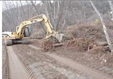
View of LWD placement within the scalloped eroded areas.
