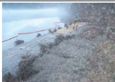
View of the erosion control fabric installation
