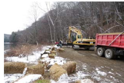
Removal of one of soil stockpiles.
