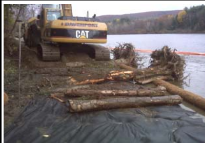
View of the root wads and log during construction of the aquatic bench.
